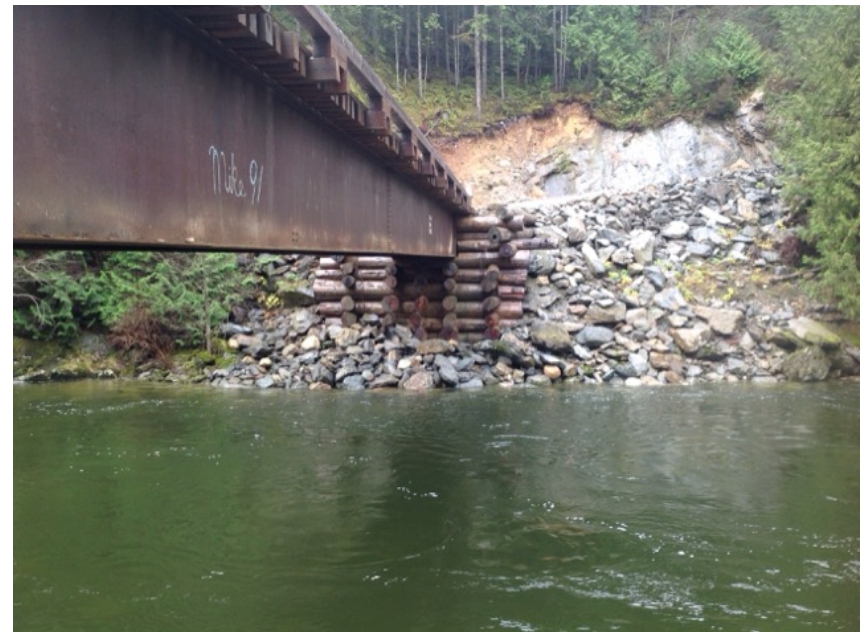
Right Bank Abutment when facing downstream
