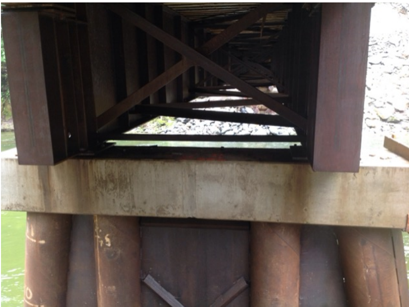
main span bearing
