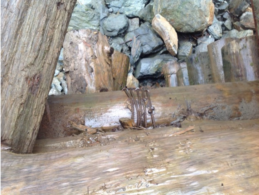
top crib log well lashed
